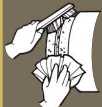
Carefully clean spigot or tongue end of pipe, including the gasket recess.
